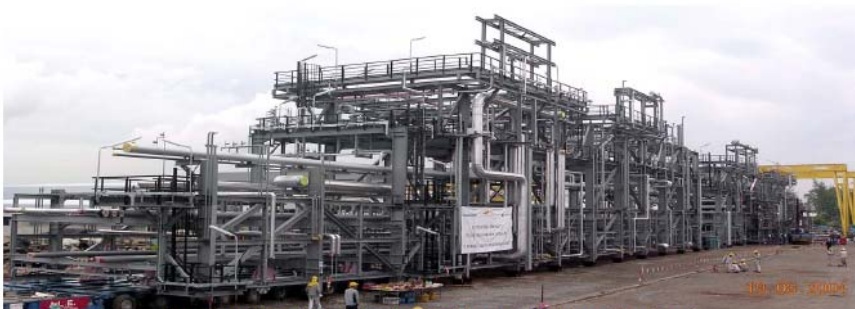
Production Module for Refinery in New Zealand
